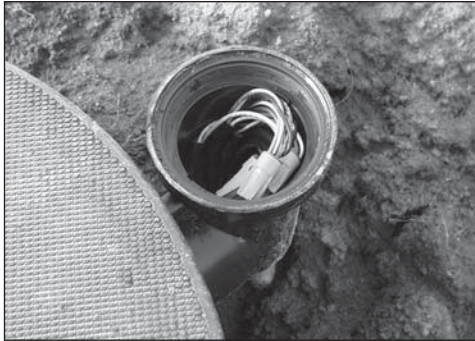
Attached outside the riser, Orenco's External Splice Box allows an electrician to access pump wiring without opening the riser lid.
